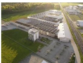
Foto 6: Belimed-Standort in Sulgen (Foto: Belimed)
